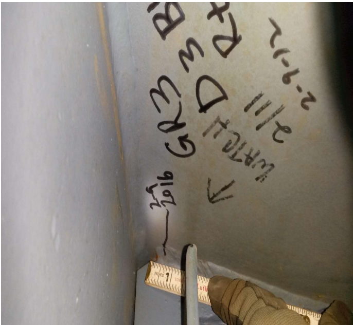
PHOTO 3 Description Girder 3 diaphragm 3 back crack in the top weld. New crack.
