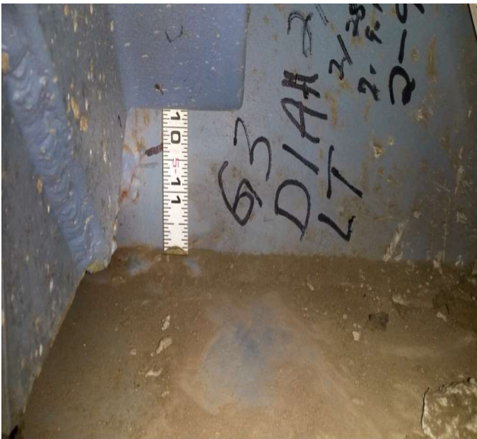
PHOTO 4 Description Girder 3 diaphragm 1 left bottom crack has propagated 1/4".
