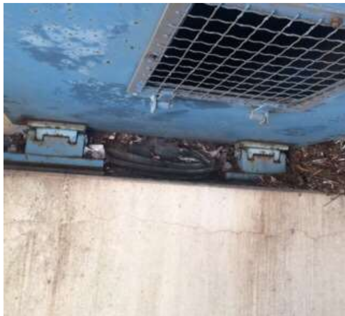
PHOTO 1 Description West abutment girder 4. Debris has accumulated on girder end and bearing due to joint seals laying on abutment.
