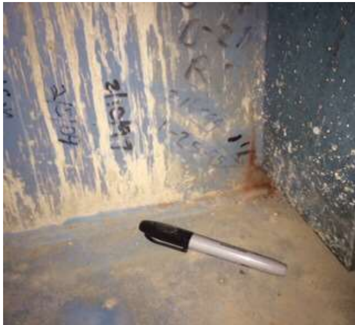
PHOTO 1 Description Girder 4 diaphragm 21 ahead crack in the web. No change.
