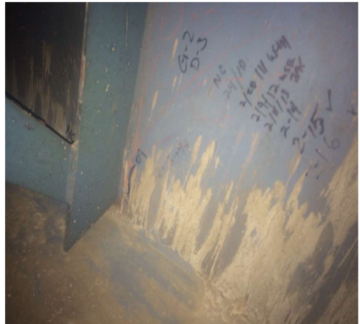
PHOTO 2 Description Girder 2 diaphragm 3 back crack in the weld. No change.
