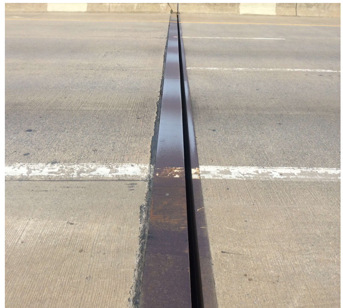
PHOTO 2 Description Bent 5 joint seal missing. Common bent .
