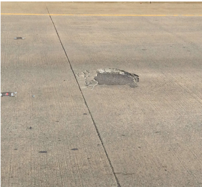
PHOTO 1 Description Span 4 spall filled with asphalt
